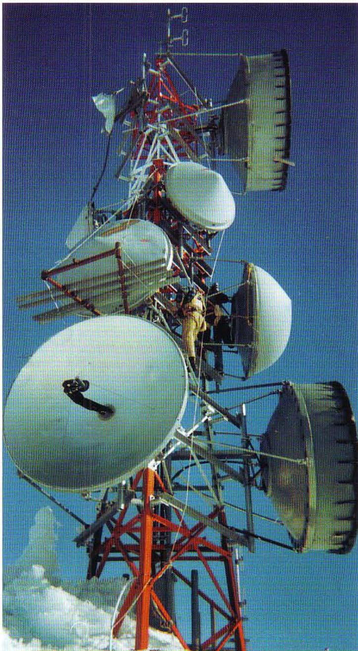
Figure 4. A microwave tower damaged by the combination of a massive ice build-up and high winds, which caused the upper antennas to break away during a storm in early March 1998. (courtesy of T. Vary, P. Eng. Varian Inc.)
